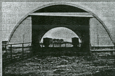
Plastic-covered hoop structures allow animals to "bed and dung" on cornstalks, straw and other materials.
